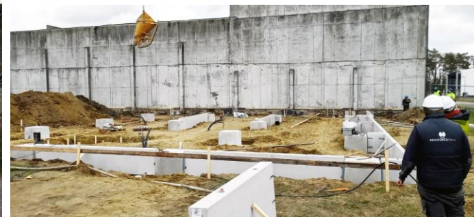
61 m 3 of foundations Kamp C, Westerlo BE (2021)
